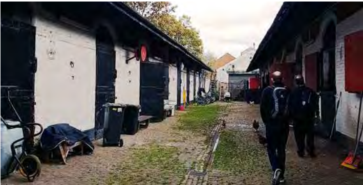
Existing stables building
