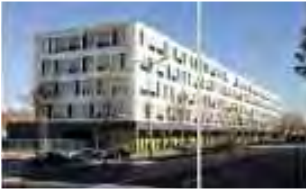
Die Gewerbehof, Laim, Munich, Germany, 2011 Situating at one of the busiest roads out of Munich and near a main train station. Five storeys, four industrial servicing/goods lifts, wide corridors and floor loading for fork lift trucks and direct servicing access to ground floor units, hosting a range of industries from robotics to food preparation.
