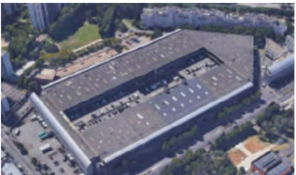
Hotel Industriel, Paris, France, 1989 Accommodating around 1,000 workspaces of various scales near Paris's orbital motorway, this three storey building has smaller units on upper floors with direct car and van access via ramps.
