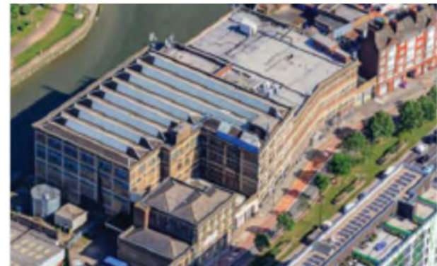
Prologis Urban Bow Yard, East London, 2019 Part Victorian, part 1930s warehouse located within a mile of the City of London and Canary Wharf, ideally placed for last mile logistics. The multi-storey building also accommodates maker spaces for creative industries including film, media, technology and storage enterprises.
