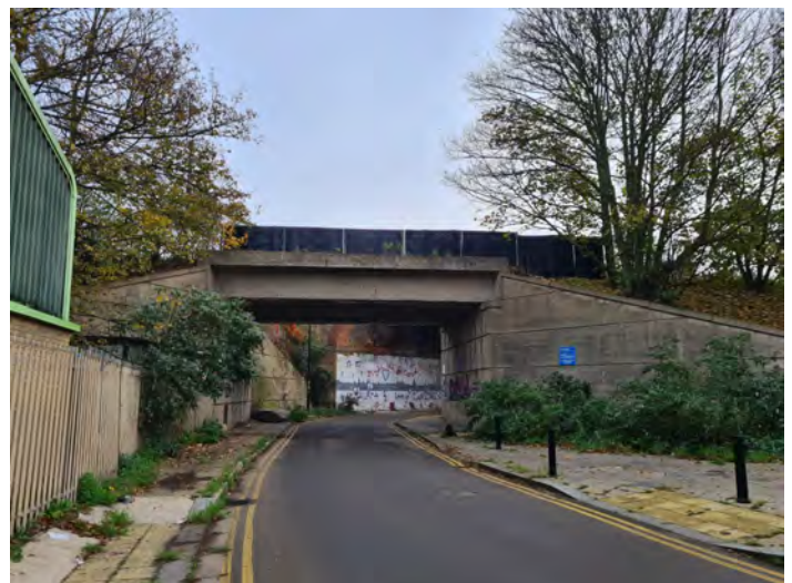
Bermondsey Trading Estate Yard
