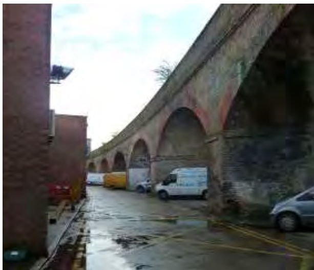
Bolina Road underpass
