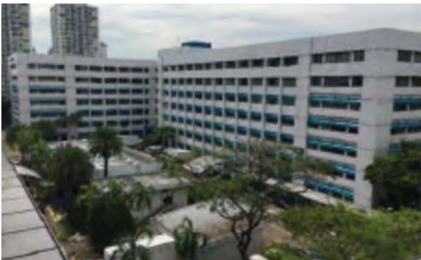
Flatted Factory – Singapore First introduced in 1960s and located close to the urban centre and labour supply, an idea pioneered in Hong Kong which accommodated low cost factory units in multi-storey buildings for the small enterprises that were a key part of the economy
