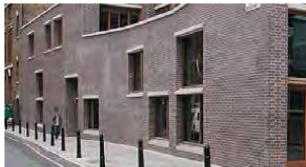
Deep window reveals and concrete lintels (Amnesty International Building - Witherford Watson Mann Architects)
