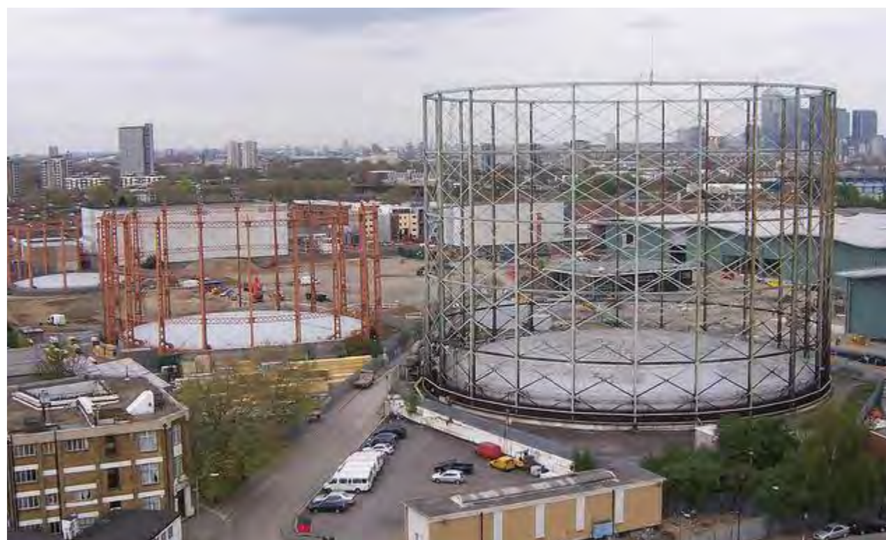
Grade II listed Gasholder No.13 (Right gasholder in picture)
