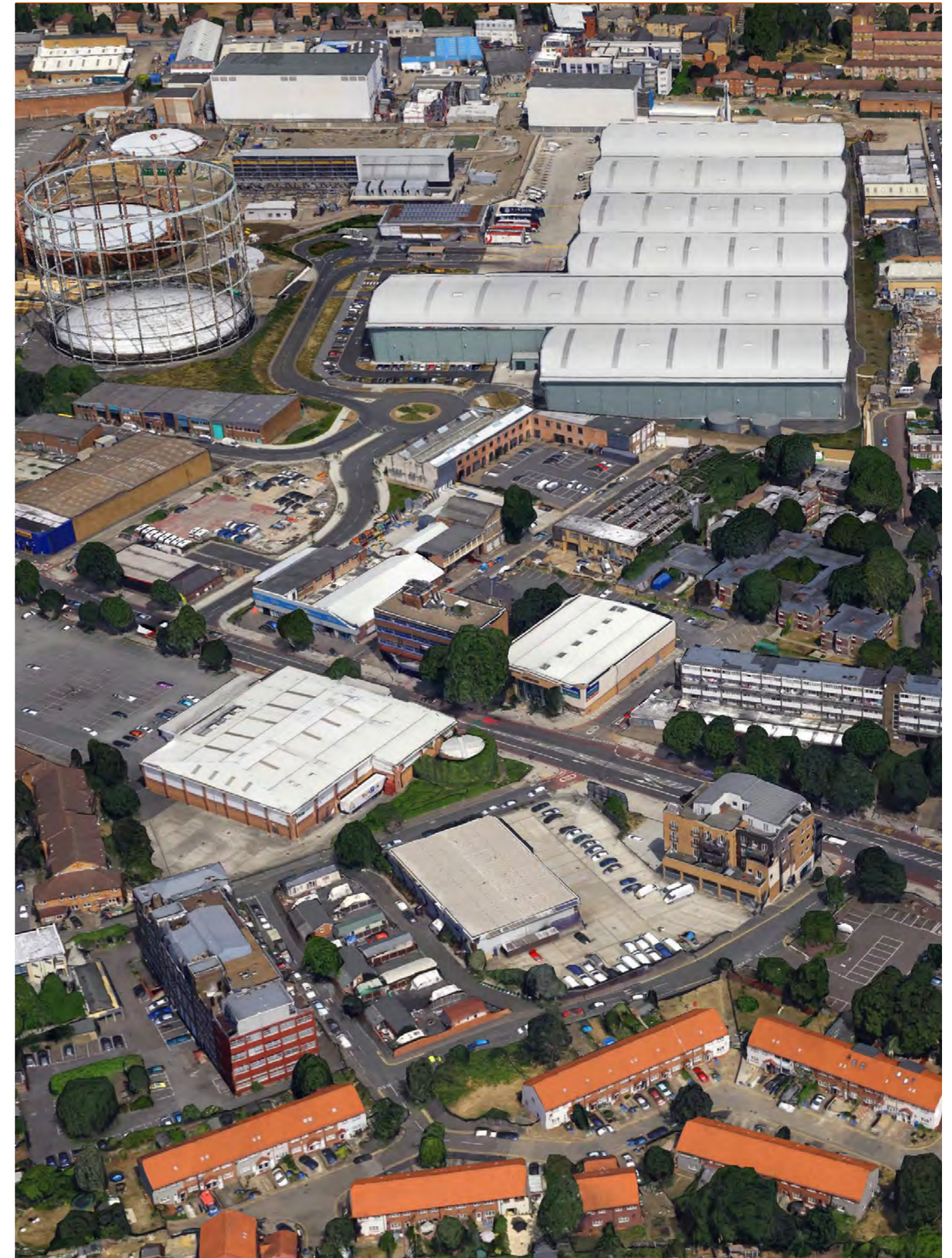
Aerial view of listed gasholder and Integrated Waste Management Facility (IWMF)
