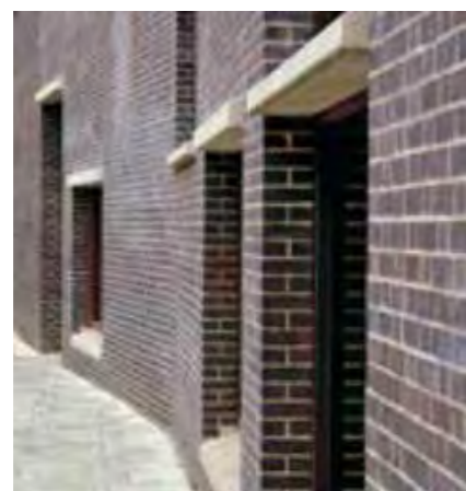
Deep window reveals with concrete lintels (Amnesty International Building, Witherford Watson Mann Architects)
