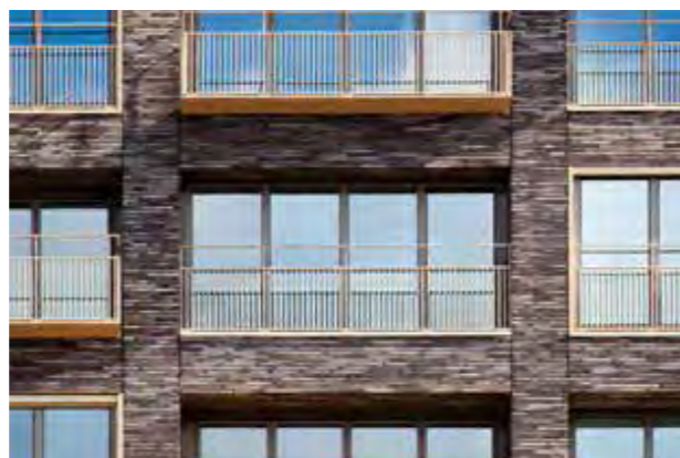
Combining glazed and regular Brickwork to manipulate light and texture(Saxon Court Housing, Maccreevor Lavington Architects)
