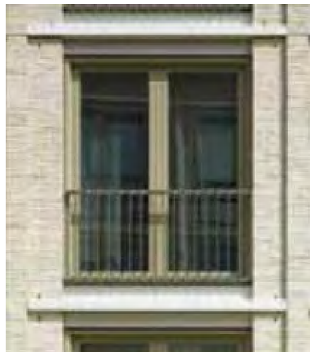
Contemporary developments illustrating the character of the architecture
