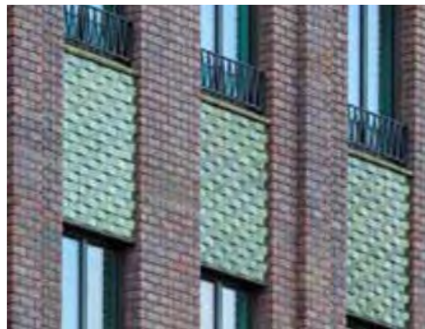
High Quality Brickwork balanced alongside delicate metalwork (Uitzicht Housing, HVDN Architecten)
