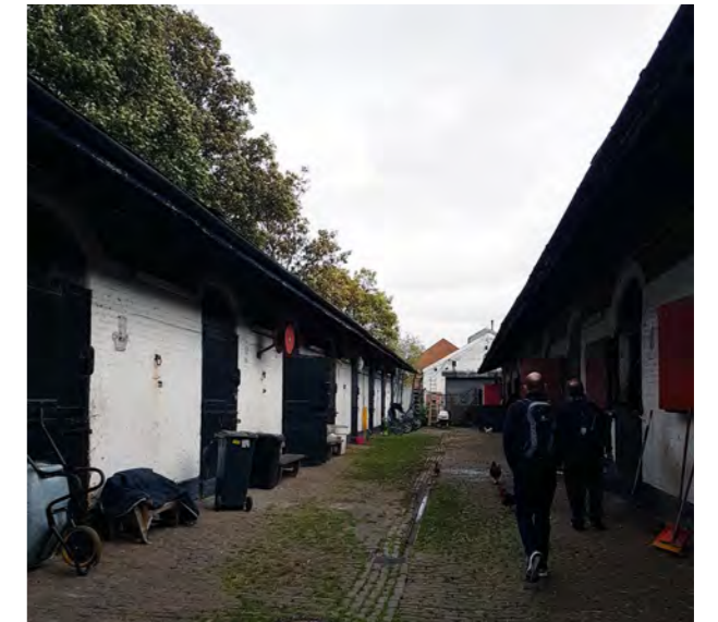
Former Southern Railway stables
