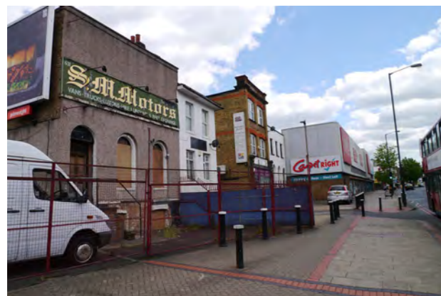
Buildings on Old Kent Road
