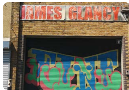
Facades with signage above ground floor doors and windows
