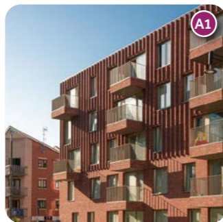
Projecting balconies to north elevations and example of texture and pattern
