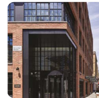
Generous glazing to ground floor shaded facades to maximize daylight and chamfered corner example
