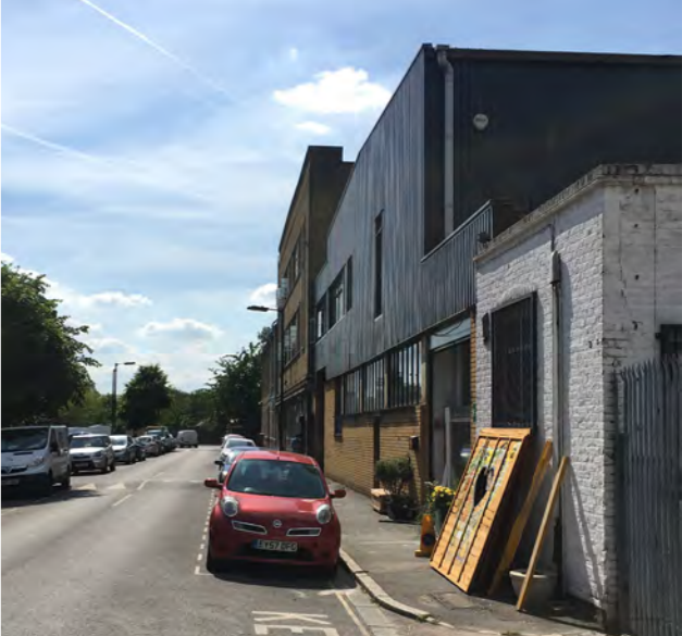
Figure 70: View of Latona Road looking west
