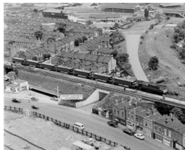
Figure 22: Historic photography of Ilderton Road
