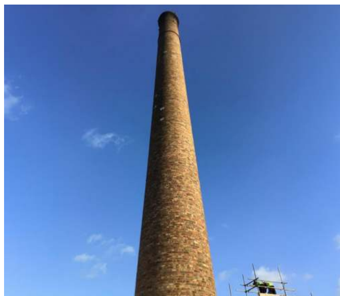
Glengall Road Chimney
