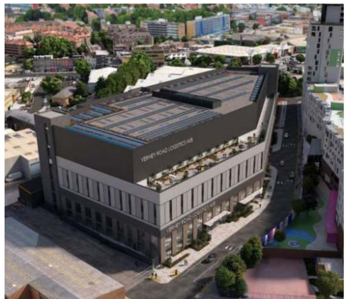
6-12 Verney Road - Stacked Logistics Hub
