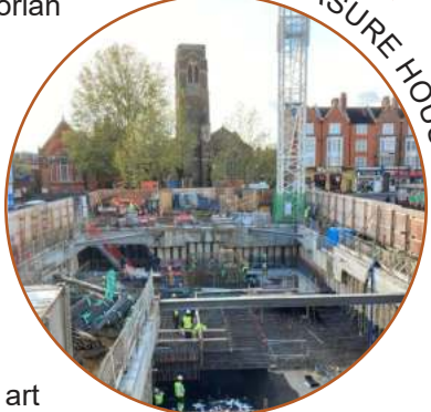
12 VIEW FROM OUTSIDE THE LEDBURY ESTATE
