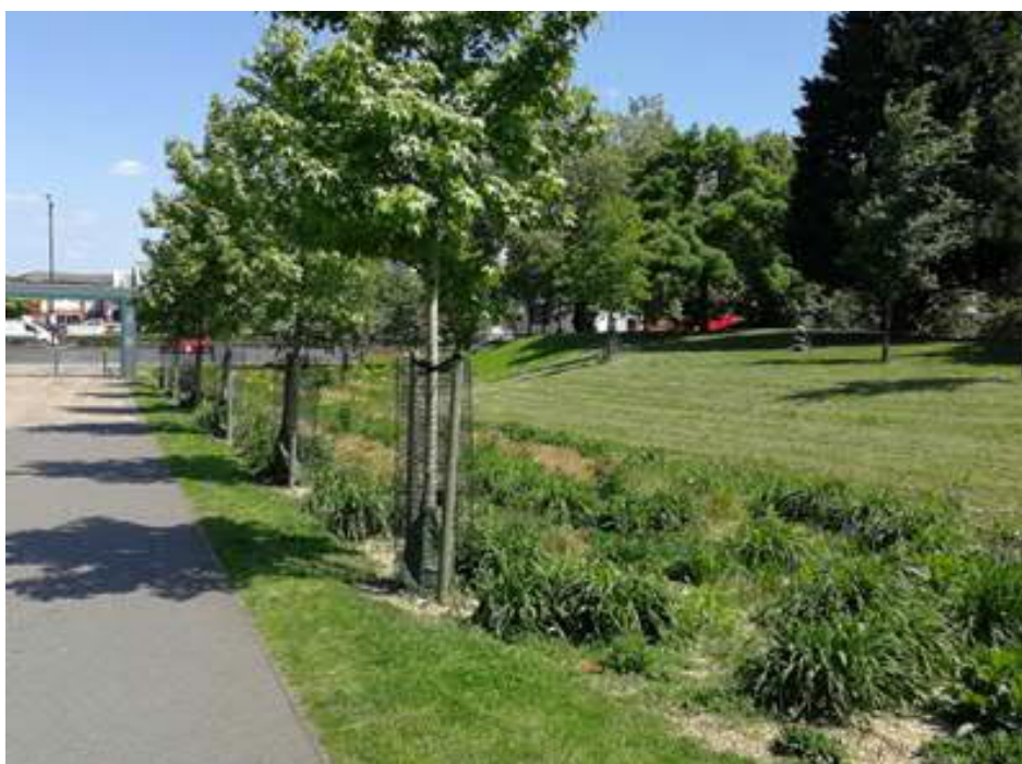
Figure 2-1: Example of existing bio-retention in the vicinity of the AAP area
