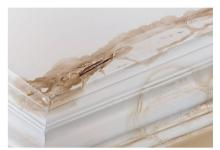
Penetrating damp is water that gets into the building from outside due to defects in the walls, roofs, windows or floors.
