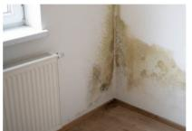
Rising damp is moisture from the ground that rises up through parts of the buildings in contact with the ground (walls and floors); it is usually found in older properties and is often misdiagnosed. It can be identified through visual inspection; however chemical testing is the most appropriate way of confirming it. Often it is due to defective damp proof courses and membranes.
