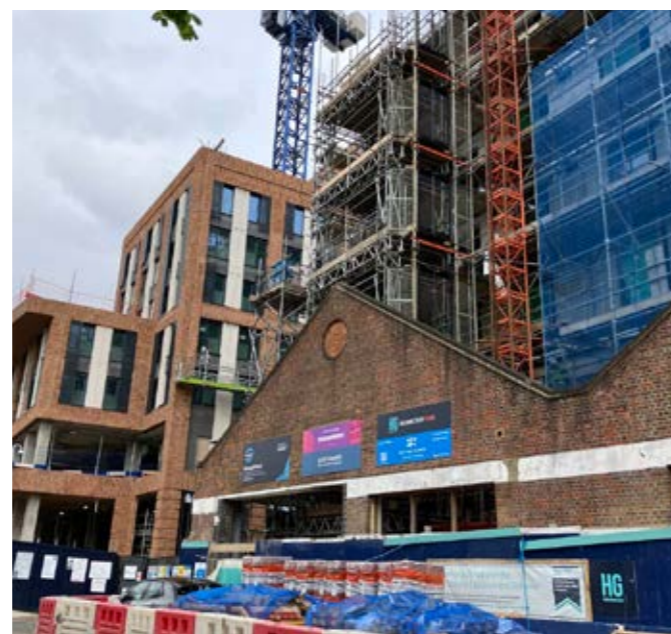
43 Glengall Road Ground and First Floor Co-Located Workspace
