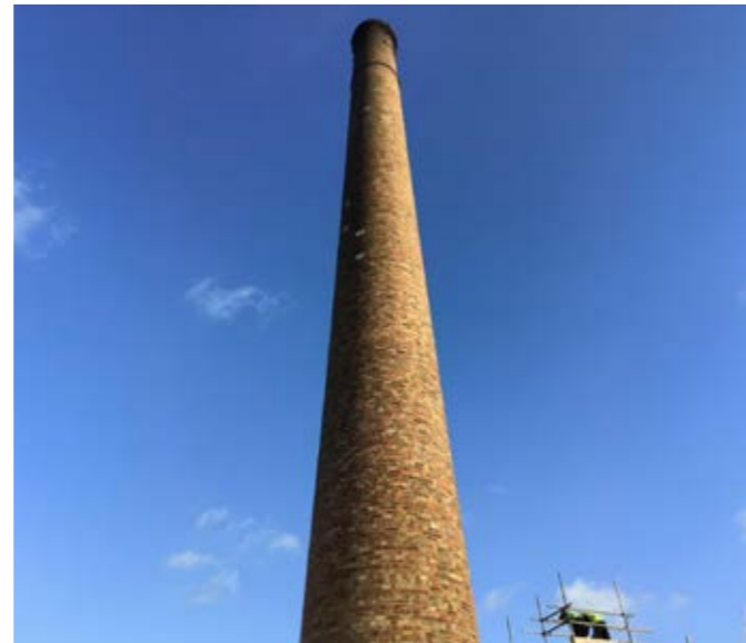
Glengall Road Chimney
