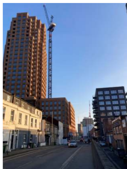
Shoulder heights along Ilderton Road
