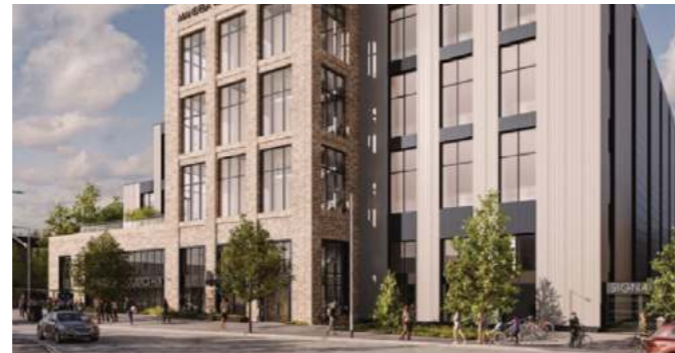
25 Mandela Way - Stacked logistics hub
