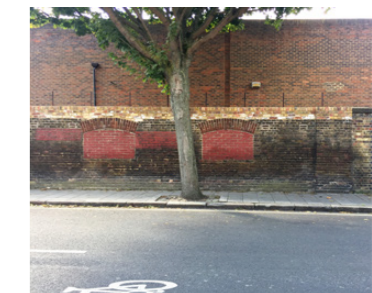
3 Brick wall is one of the few remains of Bricklayers Arms
